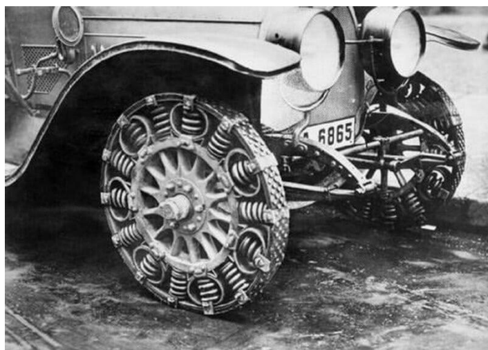
Spring steel tire on a German Protos, 1917.
